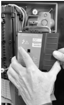
Step 5 Attach the electronics cover. Adaptor installation completed.
